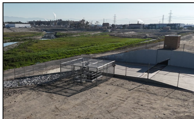
Outlet Control Gate/Rubber Dam System
